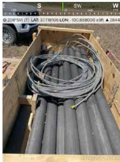
Graphite anodes ready for installation
