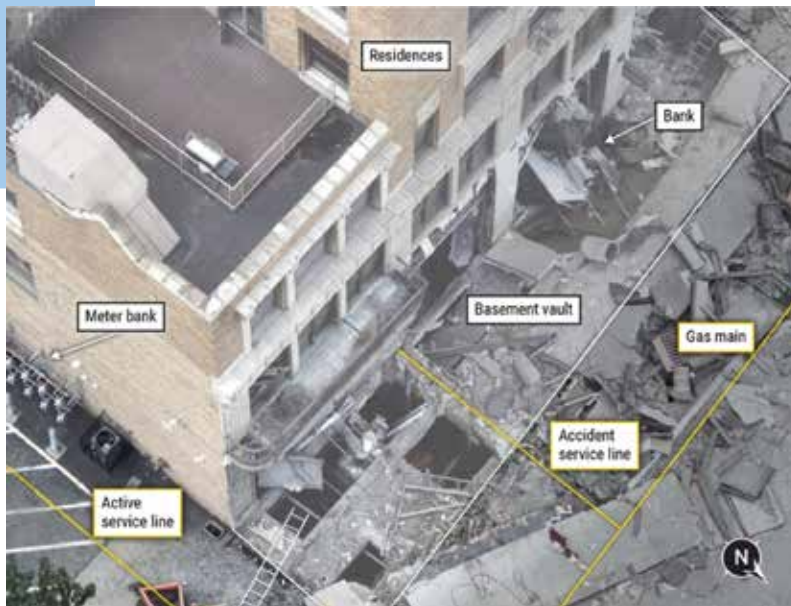
Realty building after the explosion, with approximate locations of underground assets depicted in yellow. (Source: Mahoning County Sheriff's Office)
