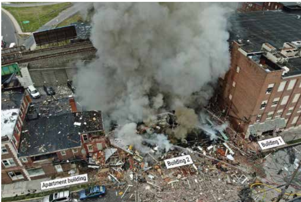
Overhead image of the accident. (Source: Western Berks Fire Department.)
