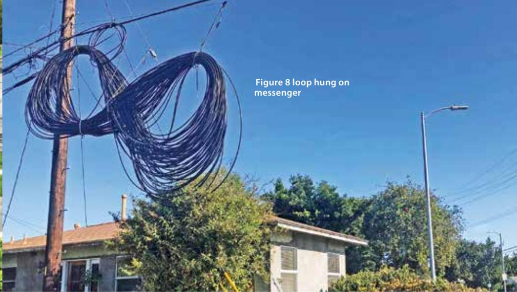
Figure 8 loop hung on messenger
