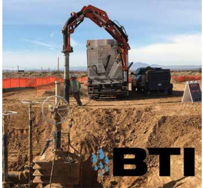
BTI owns and operates the first dry, suction excavation units in the United States, the Dino. Suction excavation provides a safer, low risk alternative to traditional excavation techniques. The Dino's high suction powered truck expertly lifts away ground, with little risk of damage to existing facilities or personal injury.
