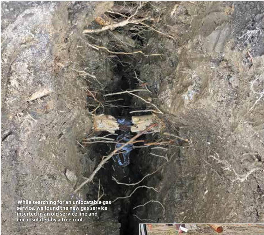
While searching for an unlocatable gas service, we found the new gas service inserted in an old service line and encapsulated by a tree root.
