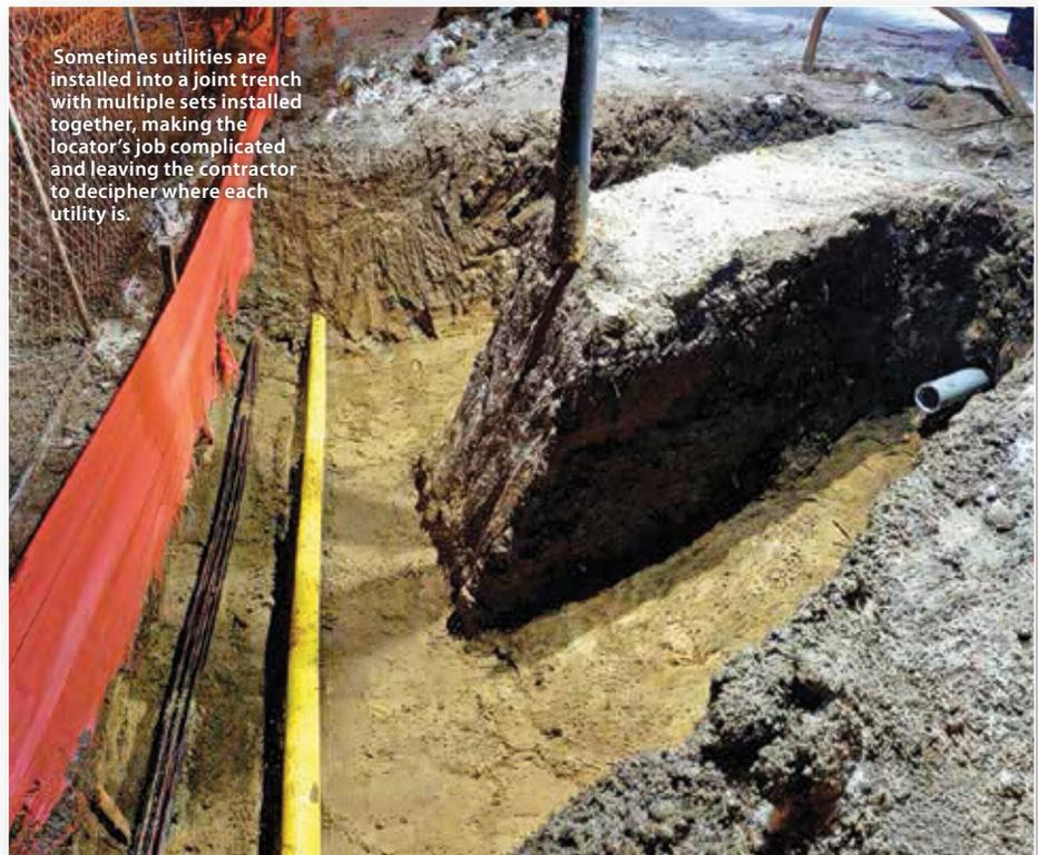
Sometimes utilities are installed into a joint trench with multiple sets installed together, making the locator's job complicated and leaving the contractor to decipher where each utility is.
