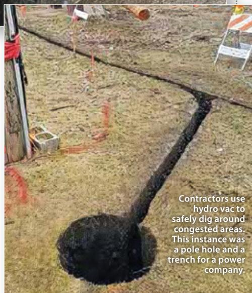
Contractors use hydro vac to safely dig around congested areas. This instance was a pole hole and a trench for a power company.
