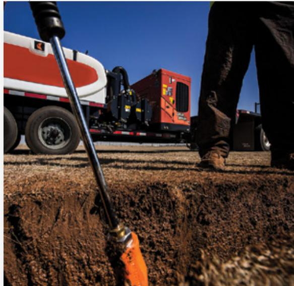
To aid in damage mitigation and keep jobsites efficient, it is vital to follow proper potholing techniques. From choosing the right nozzle to ensuring the proper water pressure, adhering to best practices in potholing can help underground construction professionals improve efficiency, increase productivity and enhance jobsite safety.
