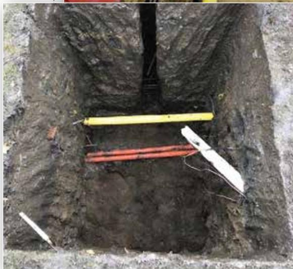
(TOP) Sometimes utilities are installed into a joint trench with multiple sets installed together, making the locator's job complicated and leaving the contractor to decipher where each utility is.
