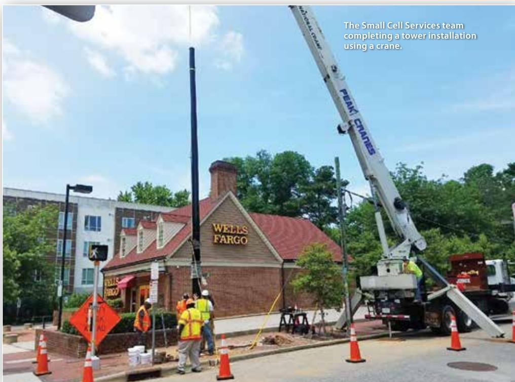
The Small Cell Services team completing a tower installation using a crane.
